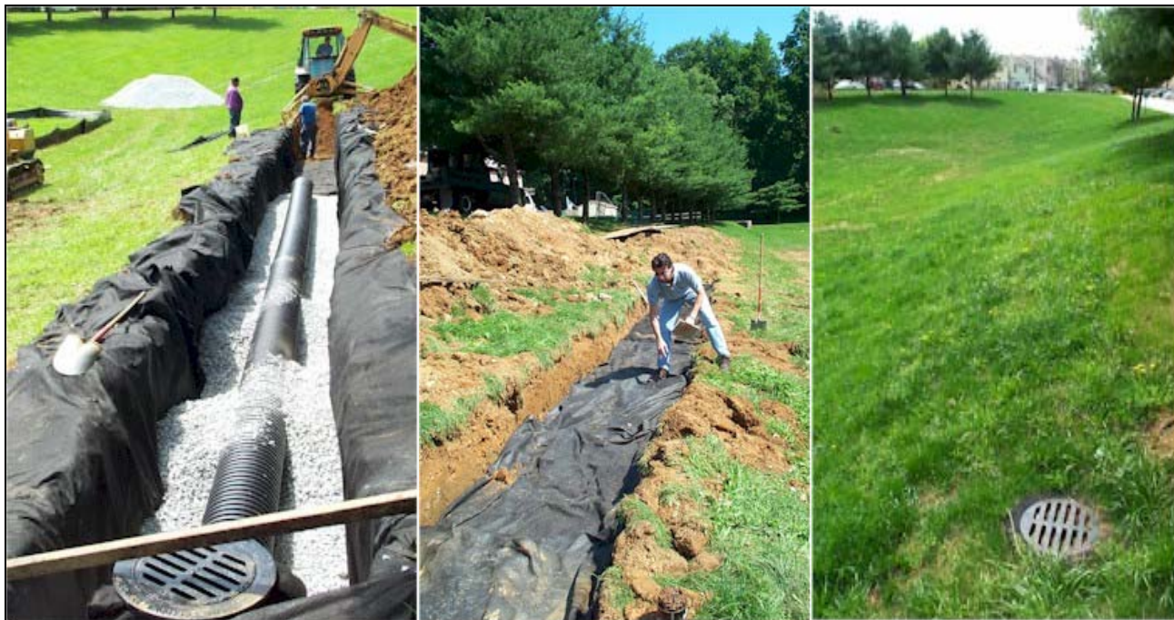
(from left to right) Installation of Inlets and Control Structure; Non-woven Geotextile is folded over Infiltration Trench; Stabilized Site
